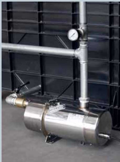
Boosting (surface pump)
